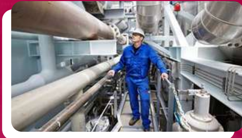
INSTALLING AND SITE SUPPORT
